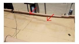
8. Evidence of ponding or pooling water on the surface of the roof.
