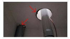
11. Lack of a fire stop noted around the heating system exhaust flu.
